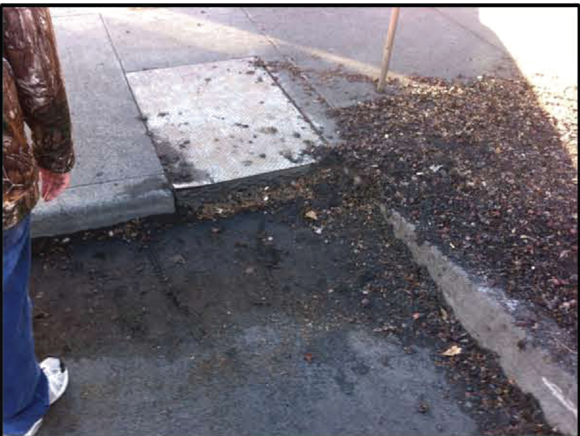
8. Drain to help water escape the parking lot during storm events. Clearly clogged and poorly managed.
