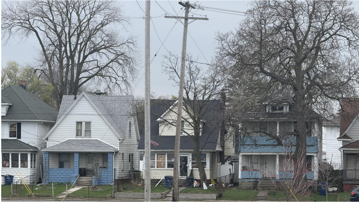
Figure 1.0. Housing directly adjacent to the Glass City Metropark. Image captured on April 10, 2026.
