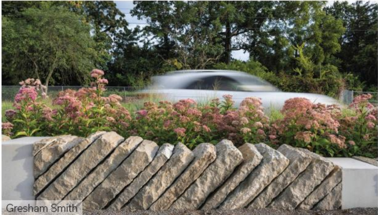
Figure 26. Signature wall detail found along Town Branch Commons composed of leaning limestone slabs set in stone dust and bracketed by pre-cast concrete wall inserts.
