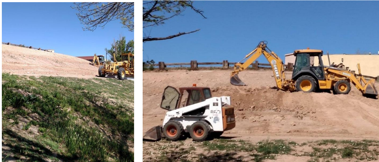
Figure 2.5 - Initial grading of the Española Healing Foods Oasis site. Heavy machinery was used to recontour the eroded slope, creating a stable foundation for future terraces, planting zones, and stormwater interventions. Images courtesy of Tewa Women United (Facebook).
