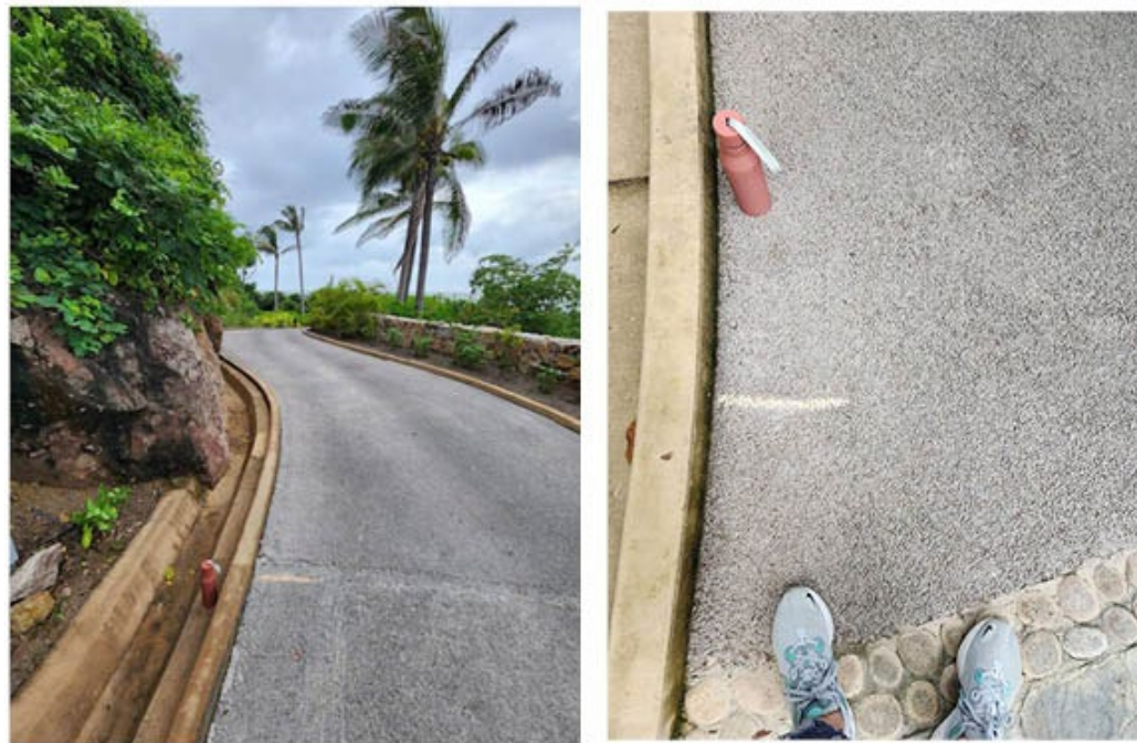
Figure 23. Photos of Focus Area 2: the golf cart path. Golf Cart Path construction material is permeable poly pavement.
