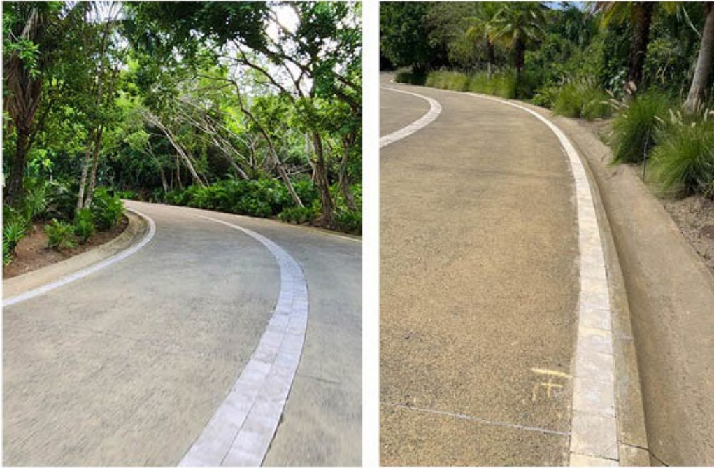
Figure 22. Photos of Focus Area 1: the surrounding access road. The Access Road construction material is permeable concrete.
