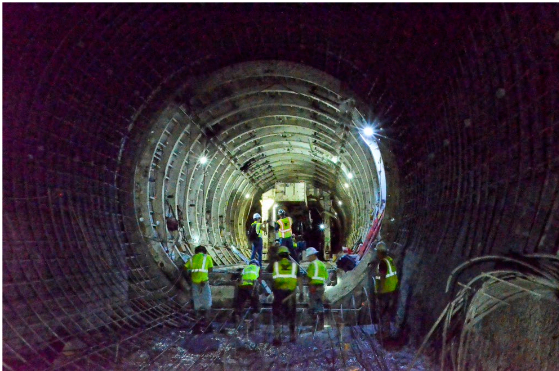
Figure a. Waller Creek Tunnel construction: Allan Shearer
