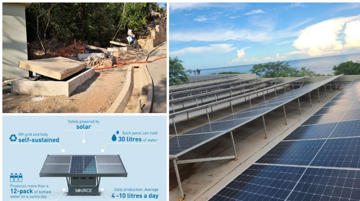
Figure 25. Overview of the Hydropanel system. Source: EDSA
