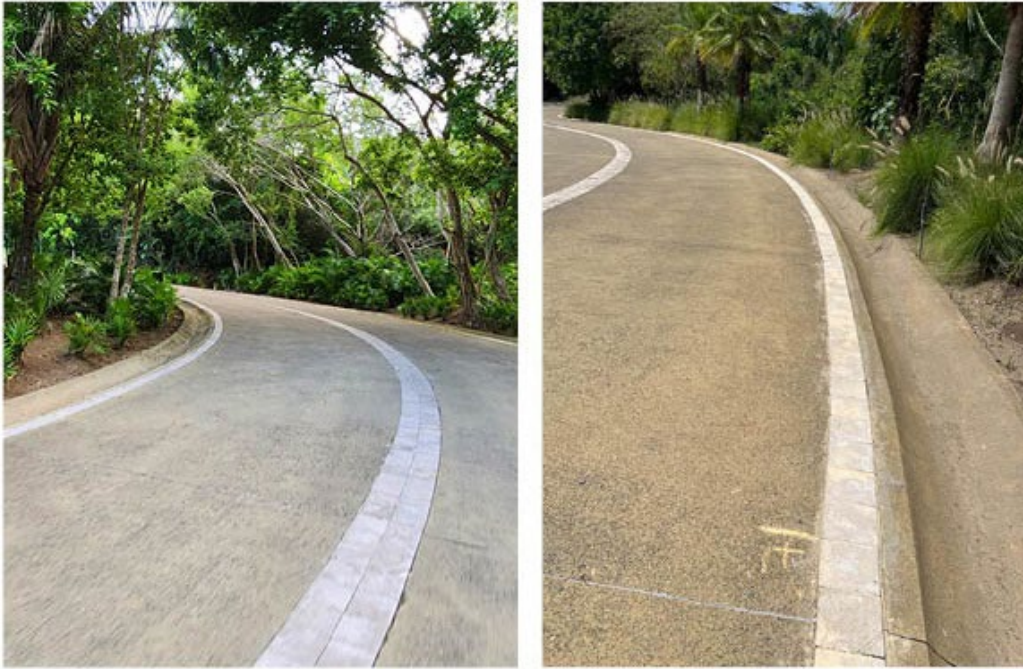
Figure 11. Photos of Focus Area 1: the surrounding access road. The Access Road construction material is permeable concrete.
