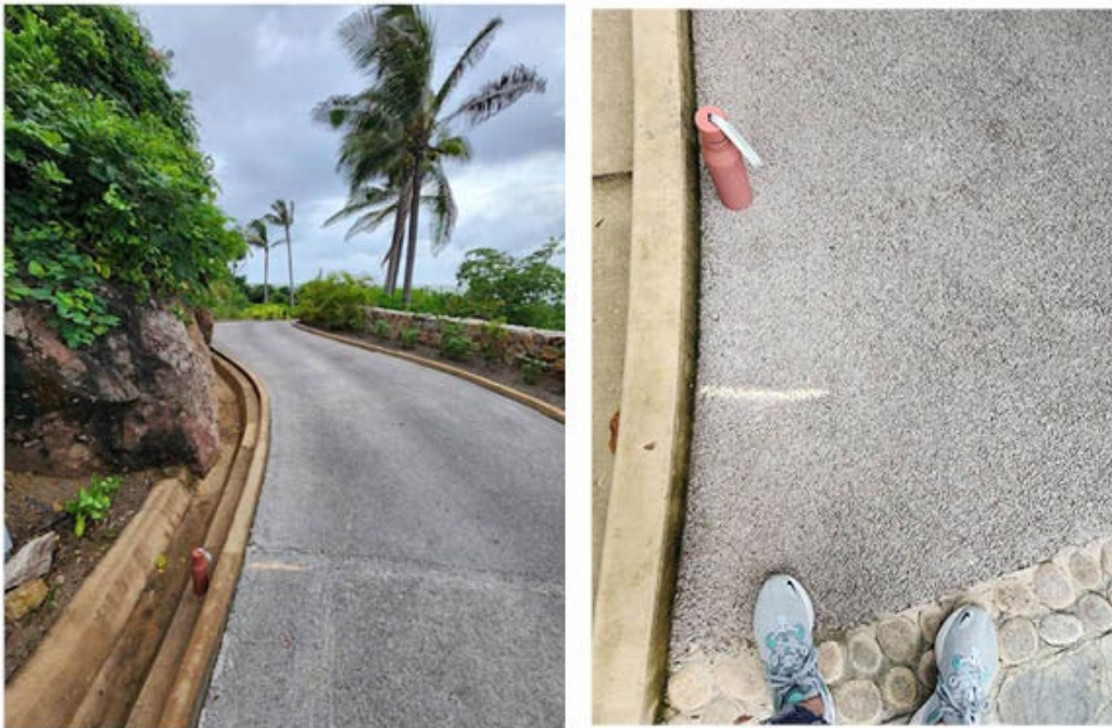
Figure 12. Photos of Focus Area 2: the golf cart path. Golf Cart Path construction material is permeable poly pavement.
