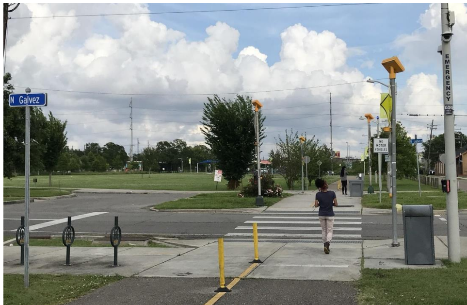
Figure 10: Lafitte Greenway pathway crossing at N. Galvez St. Traffic calming measures include crosswalk striping and solar powered rectangular rapid flashing beacons. (Photos taken by William Conrad and the LSU team.)
