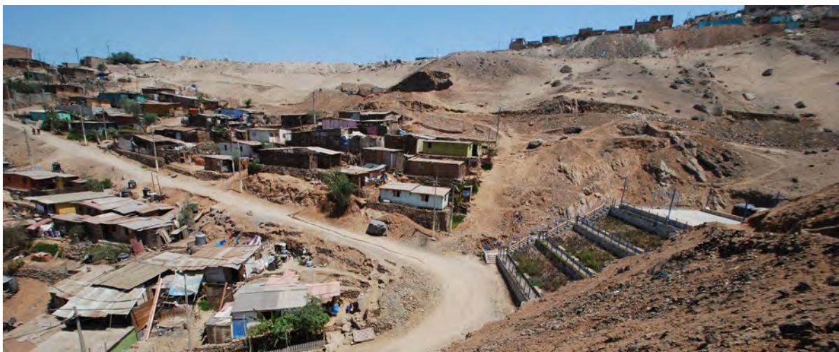
Despite significant challenges following project implementation including a two week period without water, the fog collection system, gardens and park remain in good condition. EC residents are investing their time and resources to assure the Fog Water Farms project continues to benefit the community.
