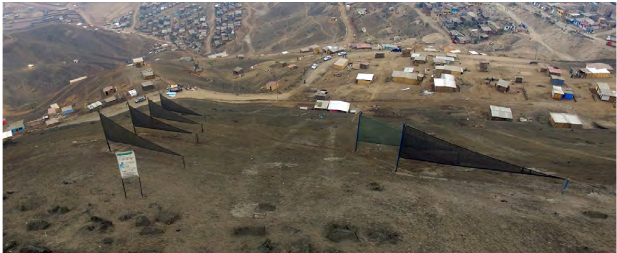
The complete fog collection system includes 6 triangular fog collectors with a combined 157m 2 of fog collection area
