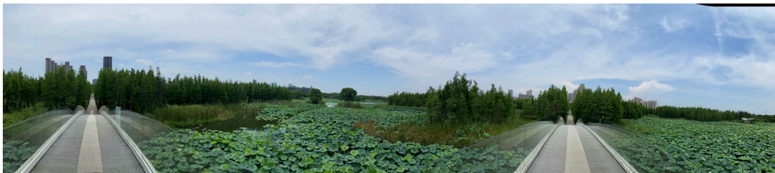
Figure 25 photo of point 16 showing raised arc bridge
