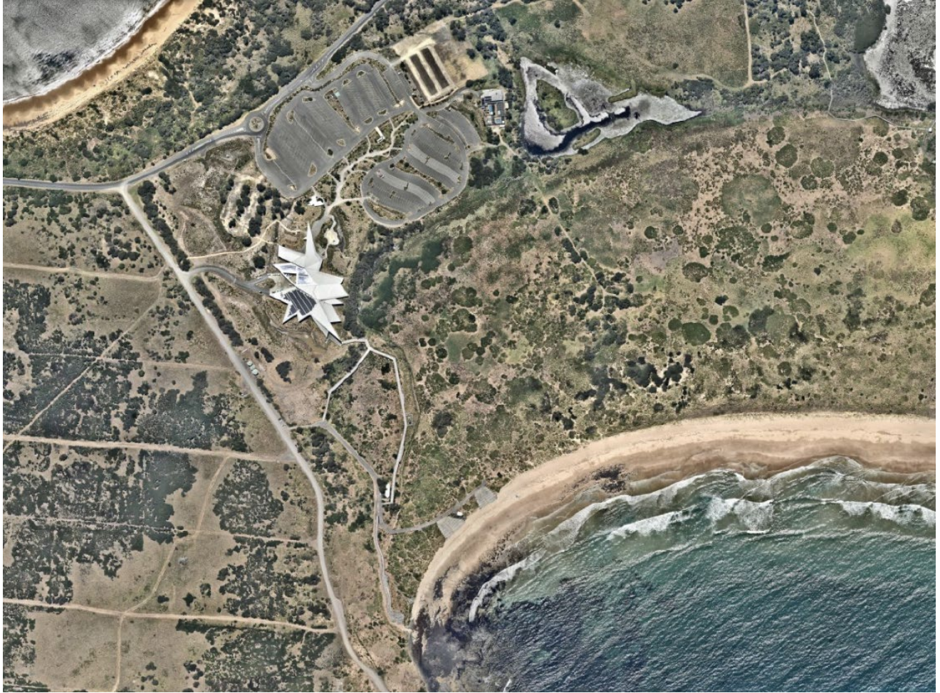
Fig. 26 Visitor centre and Penguin Parade conditions as of January 9, 2023 (Near Map aerial)
