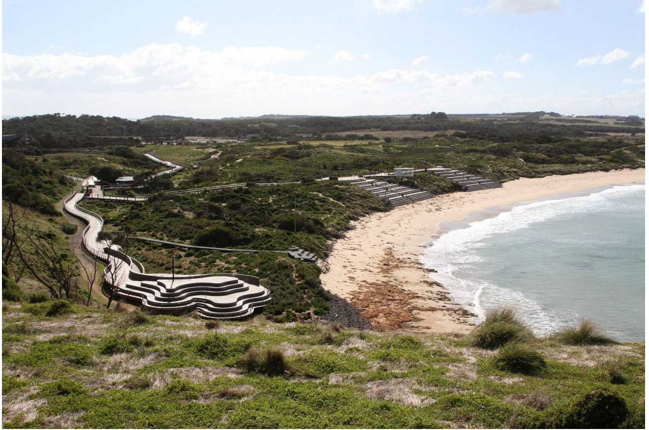
Fig. 43 Sinuous lines of the renewed Penguins Plus viewing platform and boardwalk that is responsive to the natural topography, lying lower in the landscape. To the right, a smaller viewing platform for small, guided group tours was built at the same time as the Penguins Plus. Note the new visitor centre barely visible on the top-left corner of image. (Source: Marcus Wong in https://www.flickr.com/photos/legoblock/51149420160 )
