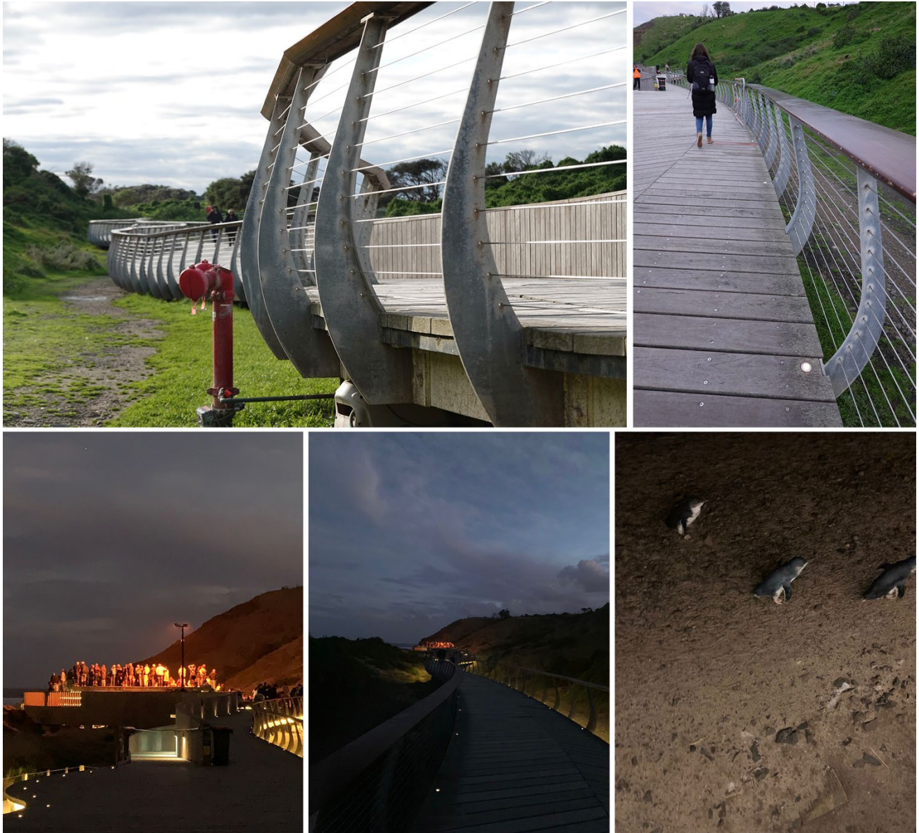
Fig. 49 Boardwalk detail and lighting strategy developed for the Penguins Plus. Compared to the previous scheme (Fig 42 and 44), artificial lighting is kept to the minimal (small uplights along the deck) – visually minimizing visitors’ presence as they walk back to the visitor centre and carpark. As can be seen in the bottom-centre image and in more detail in Fig 46 to Fig 48 above, strip lighting is integrated into recesses at the edge of the deck which illuminates the penguin’s trail (bottom-centre, bottom-right image, and beaten track in top-left image). Based on the experience at Penguins Plus, PINP has developed a lighting guideline that, for instance, requires minimal blue wavelength and zero blue spectrum emission. (Image credit: Top images by Sintusingha July 5, 2023; bottom images by Jadida March 4, 2023)
