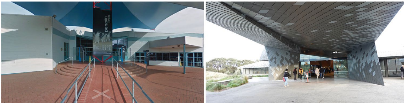
Fig. 33 Comparing the entries to the visitor centres in 2014 (Google Streetview July 2014) and in 2023 (July). Each building reflects its time. The new visitor centre, mimicking its natural surrounds, adopts a neutral grey skin that camouflages in the landscape with abstracted geometries that evoke the penguin's physical characteristics.
