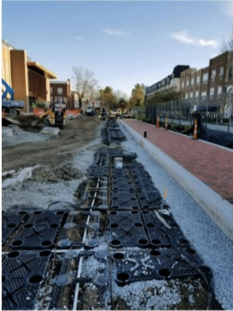
810 3X Silva Cells installed within the Monon Greenway.
