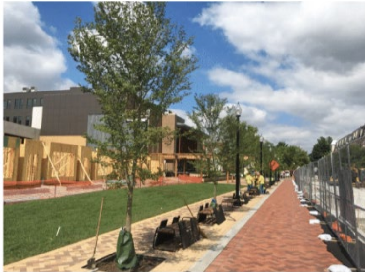
Over 140 trees planted in Silva Cells in the Monon Greenway. Tree photographed were planted in the first planting phase of 2018 .
