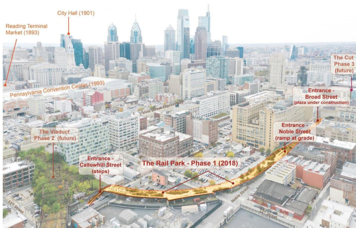
Figure 1: Oblique view of The Rail Park Phase I in Philadelphia, PA.
