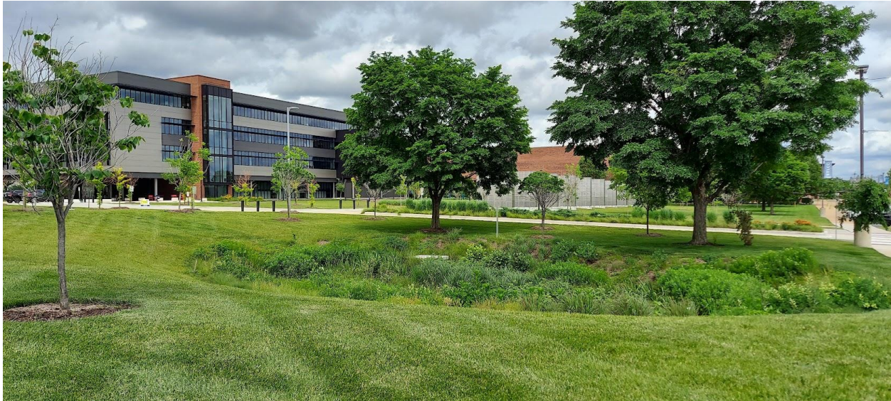
Figure 1. One bioretention basin in the renovated landscape.
