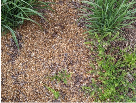
Fig 10. The 3/8" Meramec gravel cover in the bioretention garden area.
